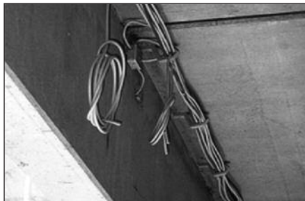
X-ECH for fastening bunched cables
